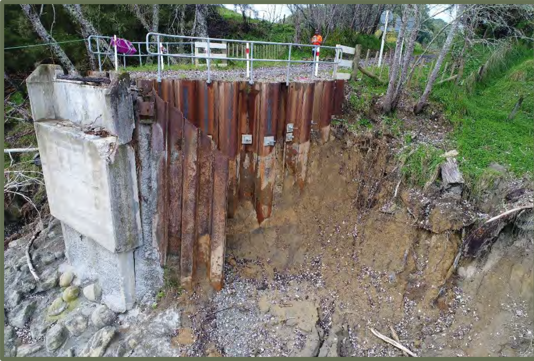
Figure 2-6: Current abutment east.
