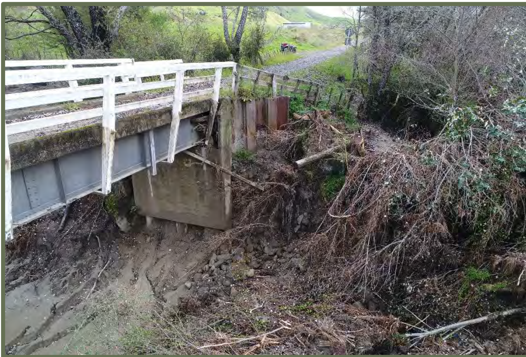
Figure 2-5: Current abutment west.
