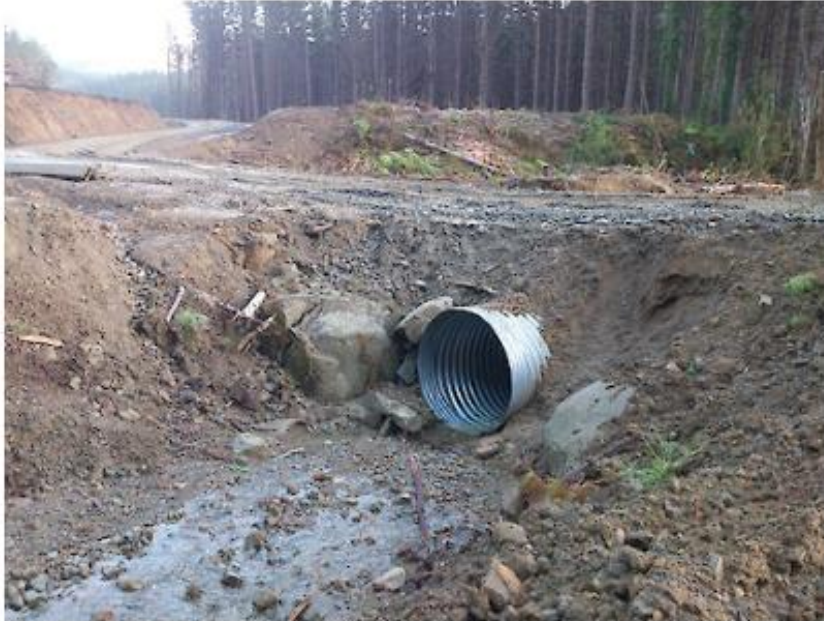
Image 1: Example of a single culvert laid perpendicular to the road and ensuring natural waterflow is maintainable. (Image reference: s8.5.1 NZFOA NZ Forest Road Engineering Manual).
